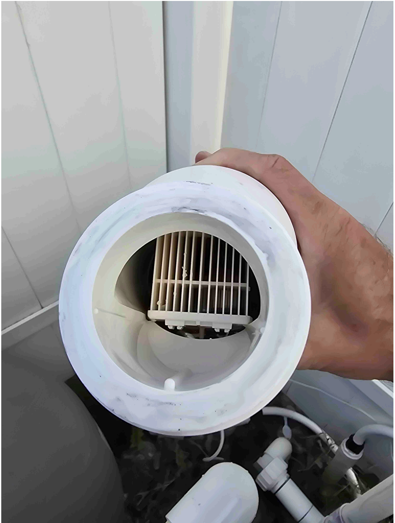
cleaned and inspected
